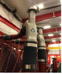
Previous attempts at coolant filtration were only effective with partial flow. OEI's design allows for full flow which exposes the coolant to a significant surface area of the magnetic field thereby capturing more contamination.
